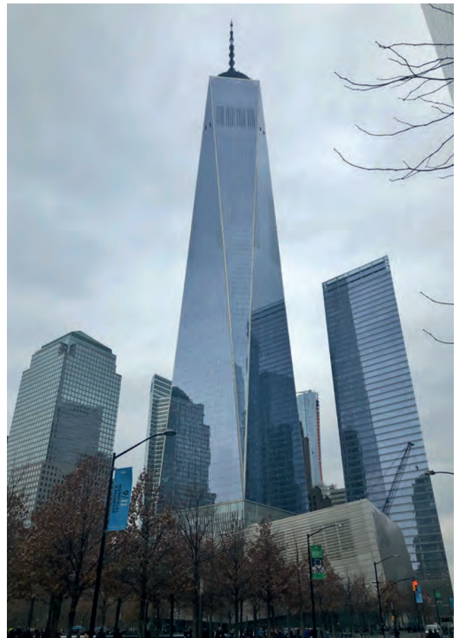
Above: At the super-skinny 432 Park Avenue in New York, a 111MPa mix enabled a height-to-width ratio of 15:1 Right: 100MPa concrete was used for the core of One World Trade Center
